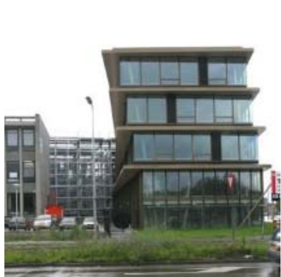
Multi-storey car-park behind existing buildings.
