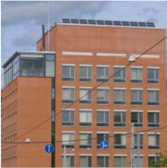
Roof-line with PV installations.
