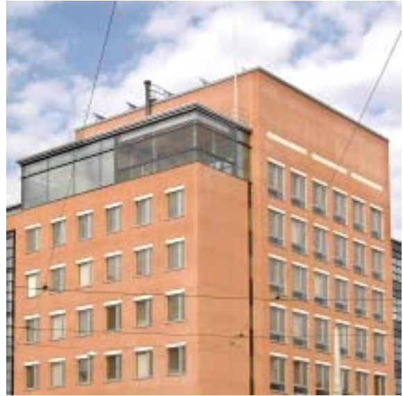
Roof-line with PV installations.
