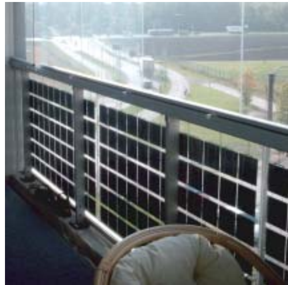
PV in balcony parapet.
