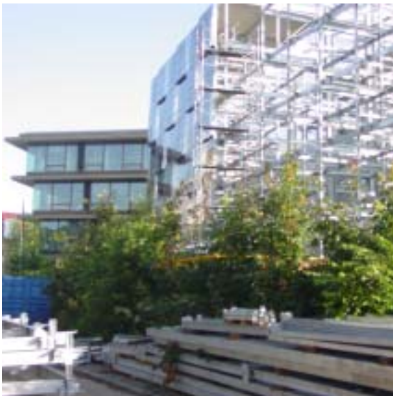
PV parking during construction.
