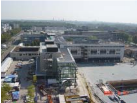
PV pergola on roof under construction.
