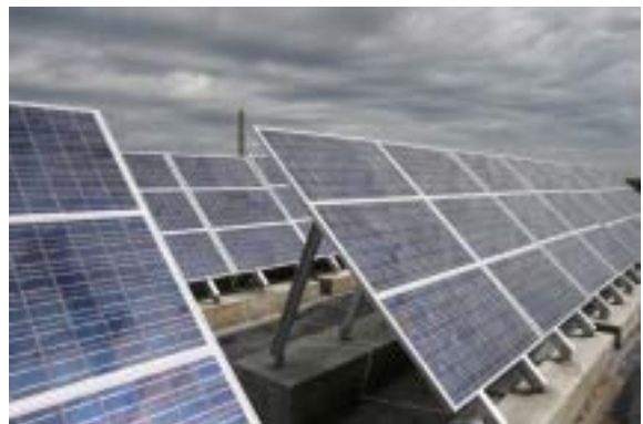
PV installation on roof.
