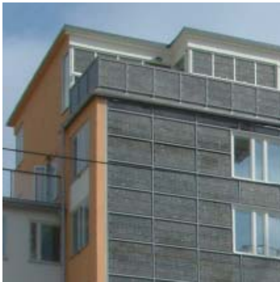
PV installation at facade, balcony parapet and windows.
