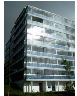
Denmark, Copenhagen PV integrated in balcony fronts
