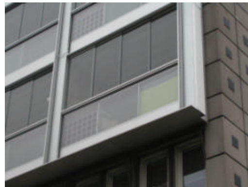
External view of a balcony.
