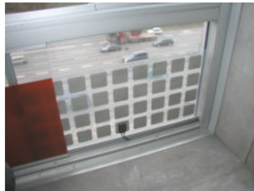
PV-module with open regulator – spring / fall.
