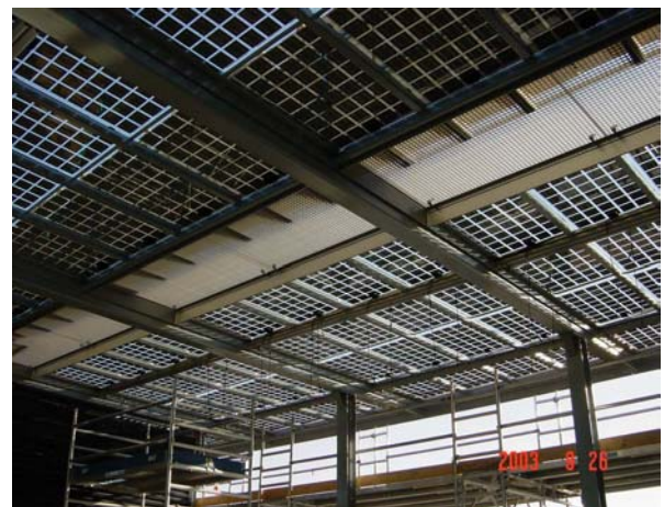
Under construction inside
