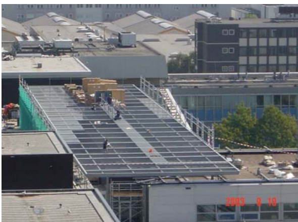
Under construction outside
