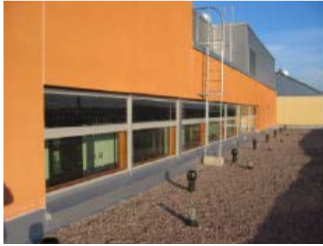
7 th floor panels (right)
